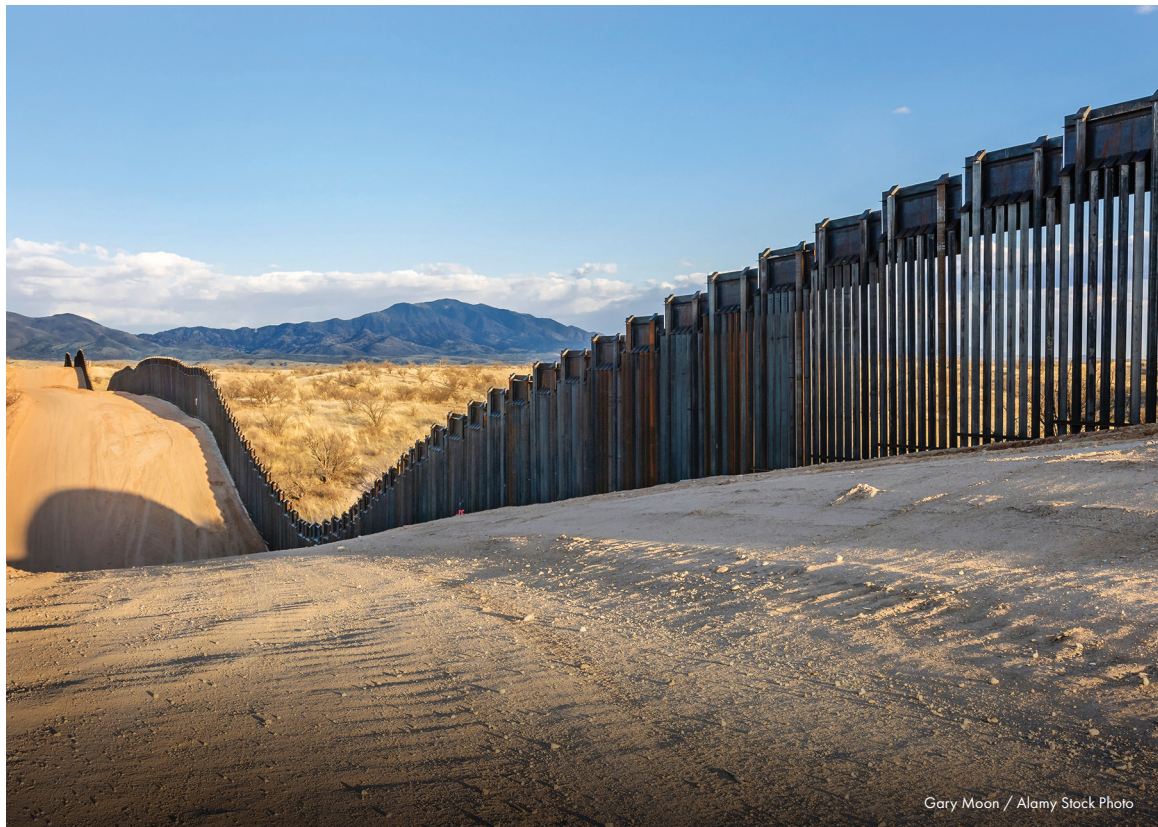
U.S. border fence east of Nogales, Arizona
