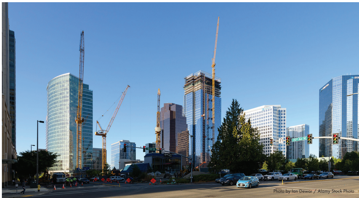
Construction cranes in downtown Bellevue, Washington (2022)
